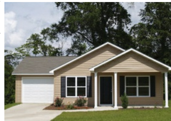
A no-step entrance, covered entryway and one-story living helps make this home age-friendly.
